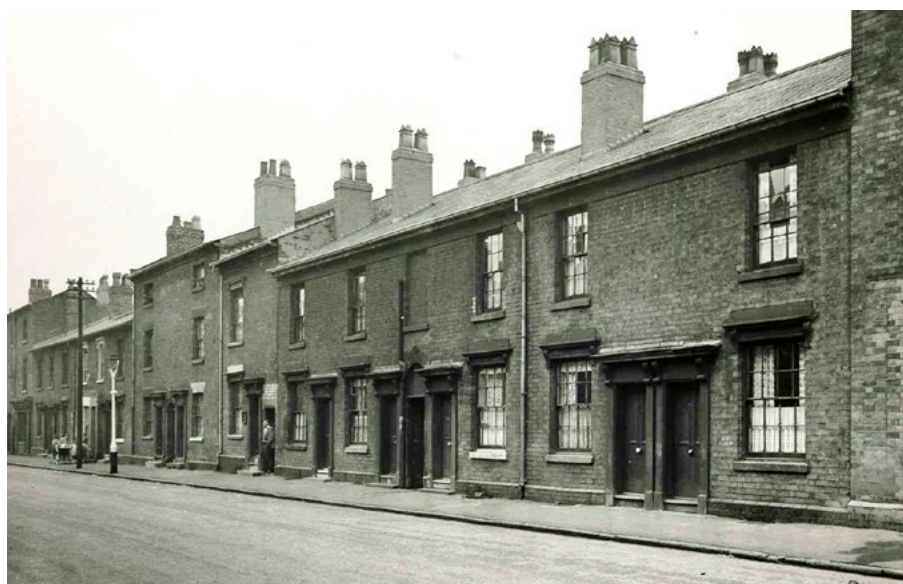
Geach Street and Geach Tower in Hockley both recall Geach the banker. Running from Summer Lane to Guildford Road, Geach Street lies just south of the Hockley Brook and the old border between Aston and Birmingham. This photo shows numbers 38-52 in the 1950s, a few years before these houses and the rest of the buildings were cleared away.
